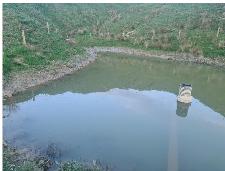
Figure 1: Sediment trap for 3.6 ha catchment
